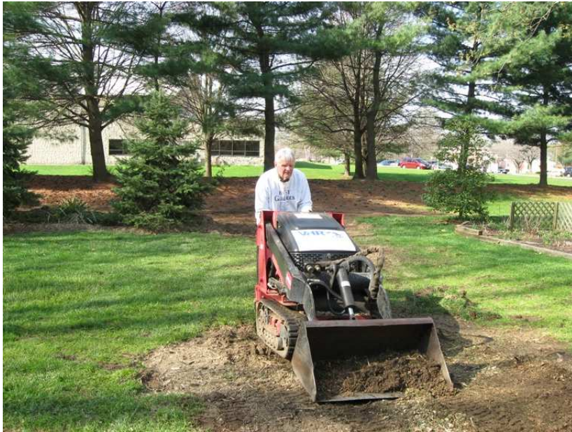
Clearing wood chips
